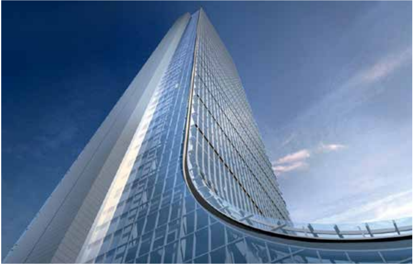
Sapphire Residence and Commercial Center Istanbul, Turkey
